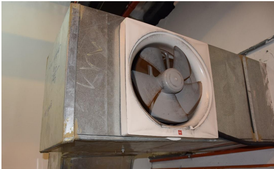
Figure 5.3.2.1 Exhaust Fan located in machine room
