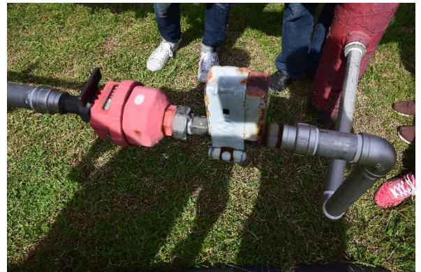
Water meter for the internal water usage
