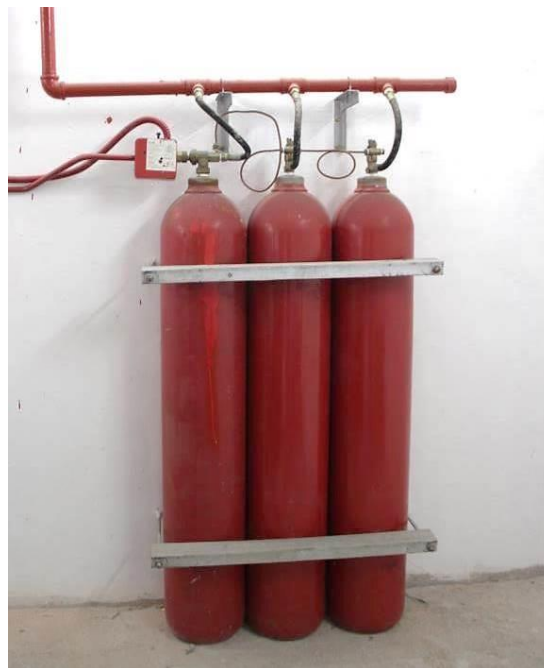
Figure 1.2.3.2.1 Carbon dioxide suppression system
