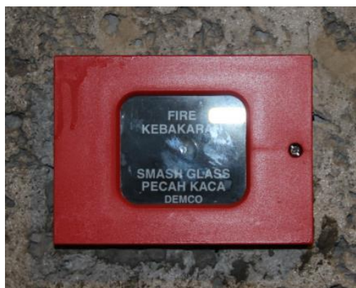
Figure 7.2.10.2.1 Manual Fire Alarm
