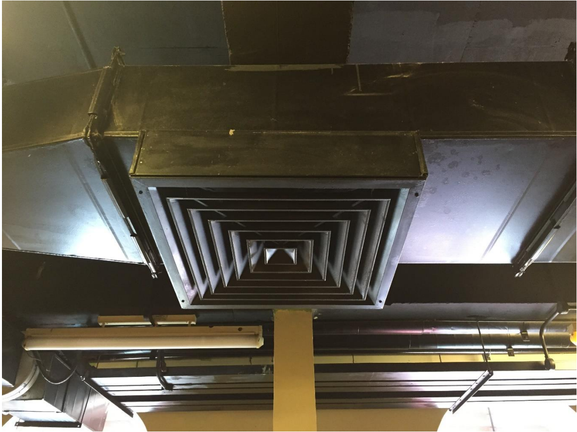
Figure 6.2.2.3.2 Fan Coil Unit Diffuser
