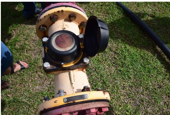
Water meter for fire fighting system
