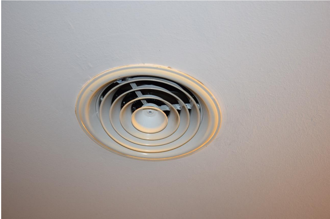
Figure 6.2.2.1.5 Ceiling Diffuser
