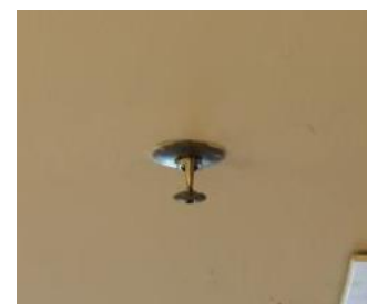
Figure 7.2.5.2.1 Sprinkler head
