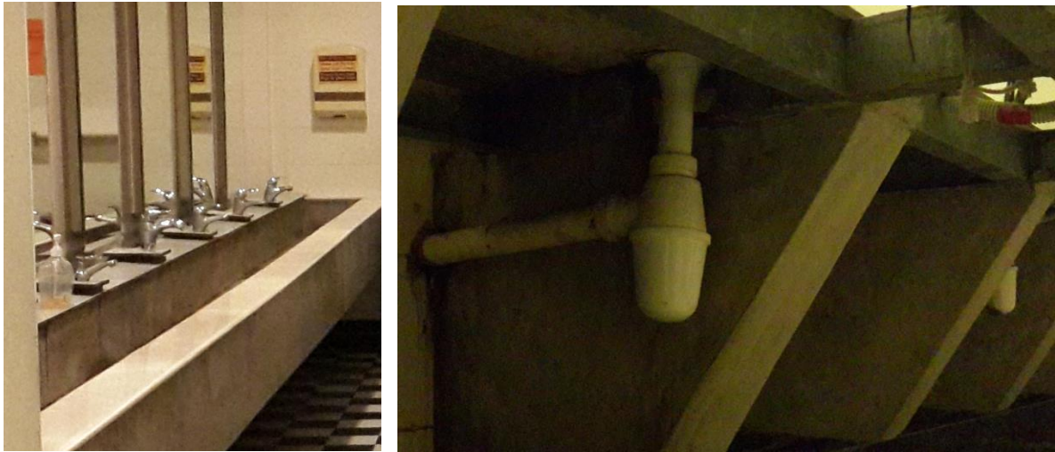
Figure 4.3.1.3.1 (a) & (b) Wash Basins and water seal trap taken in the washroom of KL Pac
