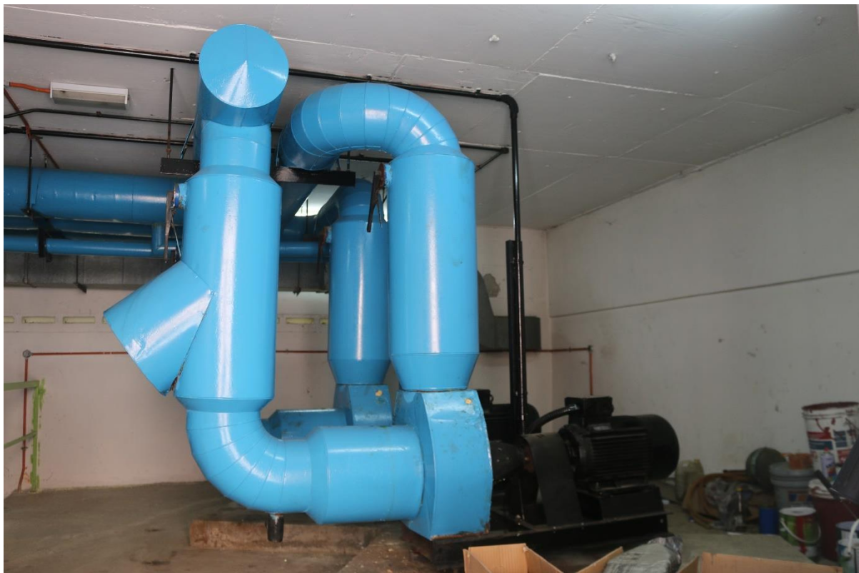
Figure 6.2.1.2.1 Condenser Water Pump with Condenser water supply pipe
