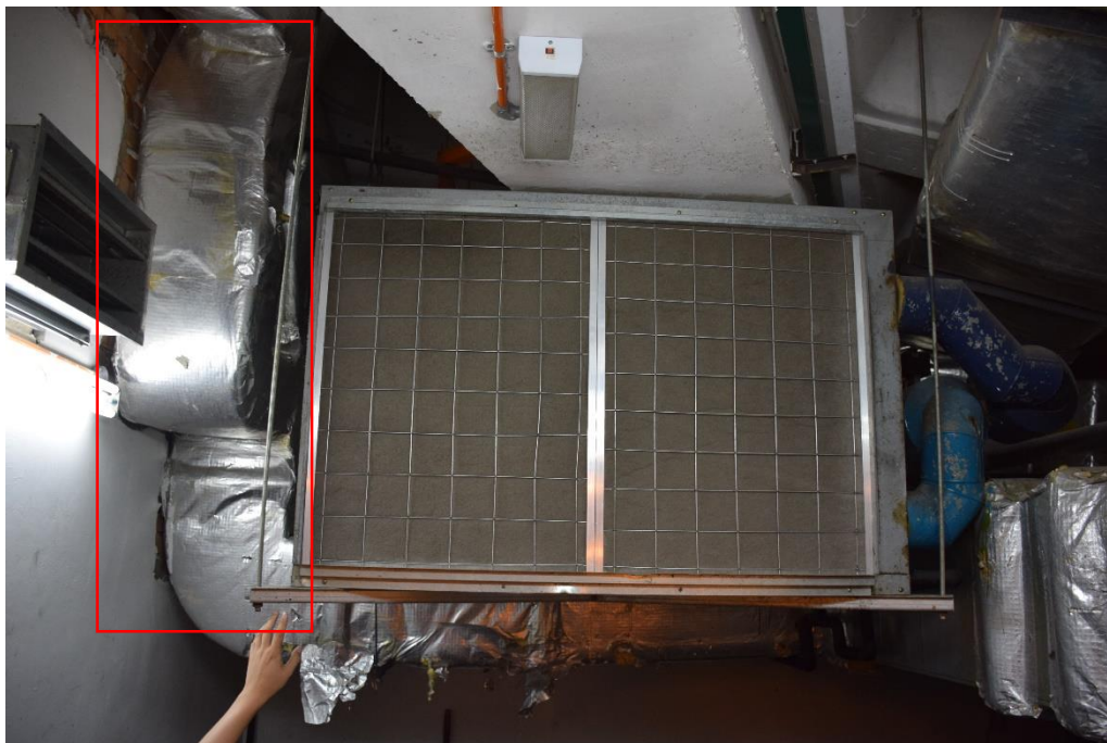
Figure 6.2.2.1.3 Sheet metal Duct System
