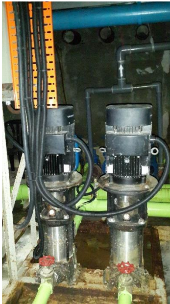
Figure 2.3.4.1 Vertical Booster Pump
