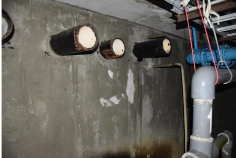
Figure 2.3.5.1 Overflow Pipes
