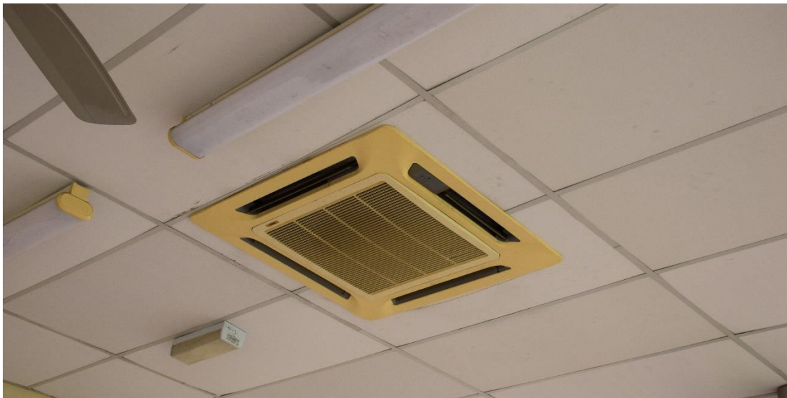
Figure 6.2.2.3.3 Fan Coil Unit Diffuser (Cassette Type)
