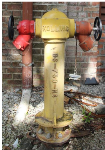
Figure 7.2.7.2.1 External Fire Hydrant
