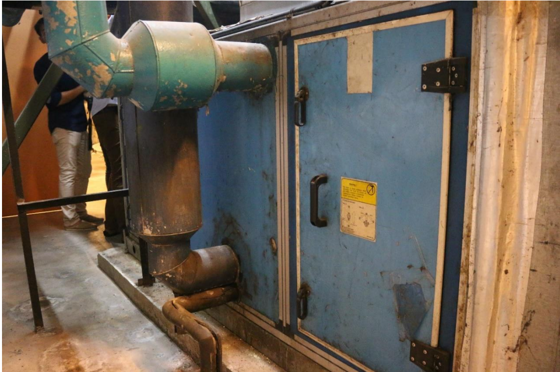
Figure 6.2.2.1.1 Horizontal Air Handling Unit with modular design
