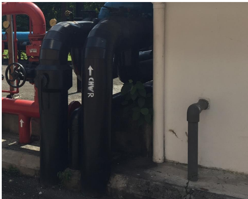
Figure 6.1.2.2.5 Chiller water Return Pipe (CHWS)
