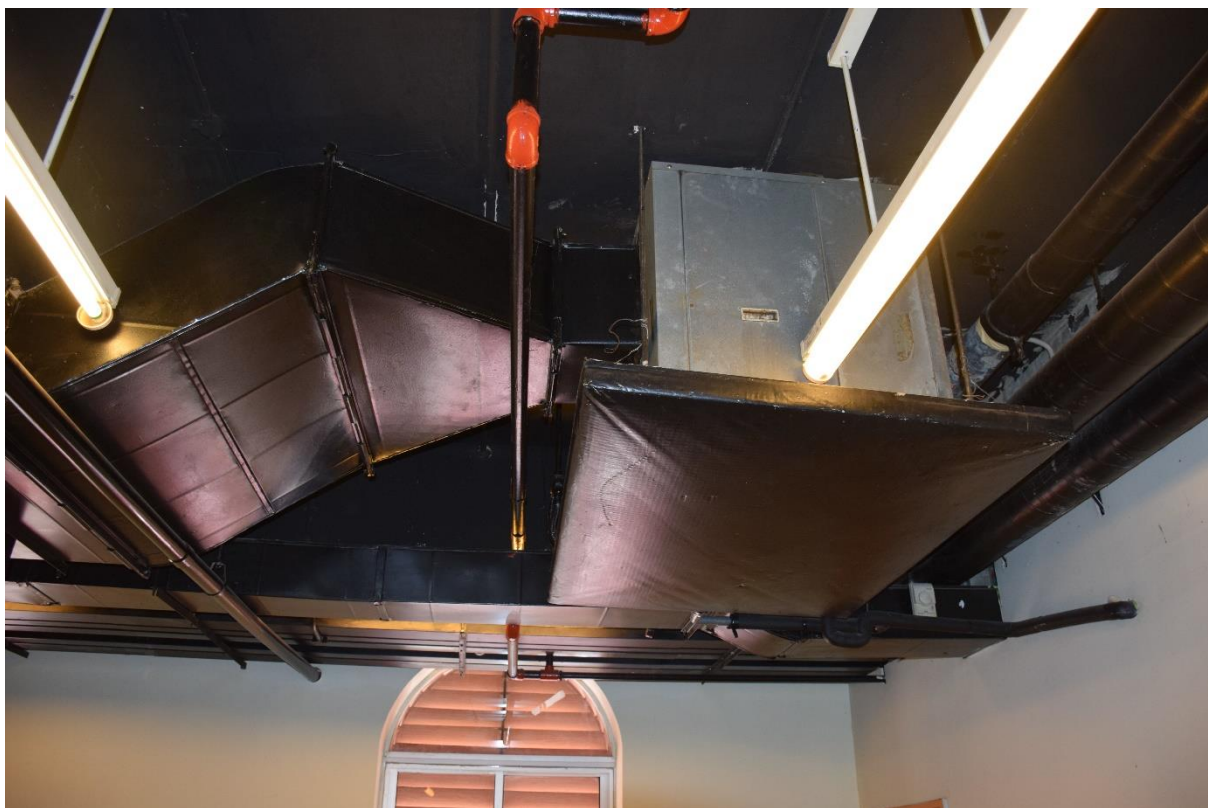
Figure 6.2.2.3.1 Fan Coil Unit
