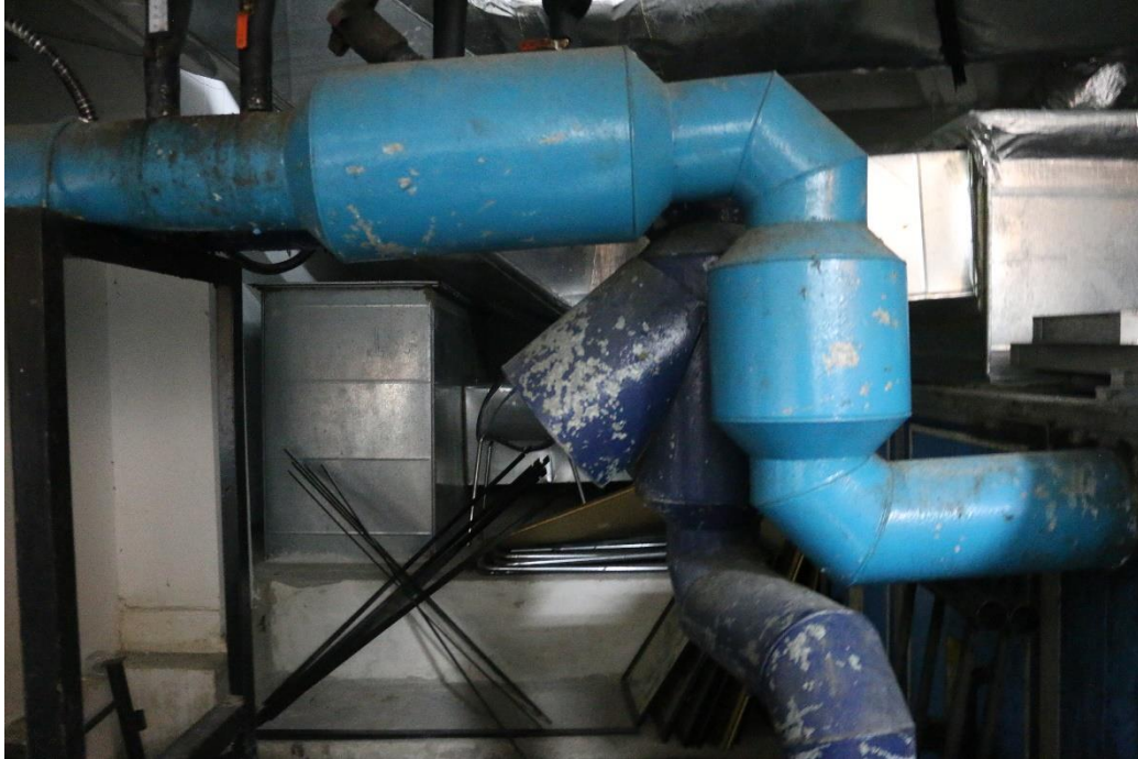
Figure 6.1.2.2.4 Chiller water supply Pipe (CHWS)
