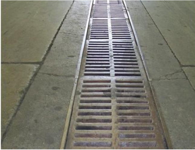
Figure 4.3.3.1.3 Perimeter Drain
