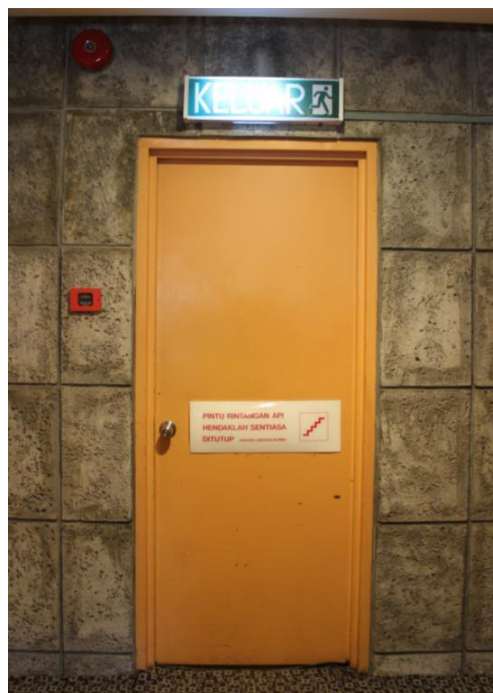
Figure 7.3.4.1.1 Fire rated door
