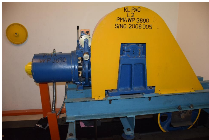
Figure 5.3.2.2 The Geared Machine on top of I-Beam Structure
